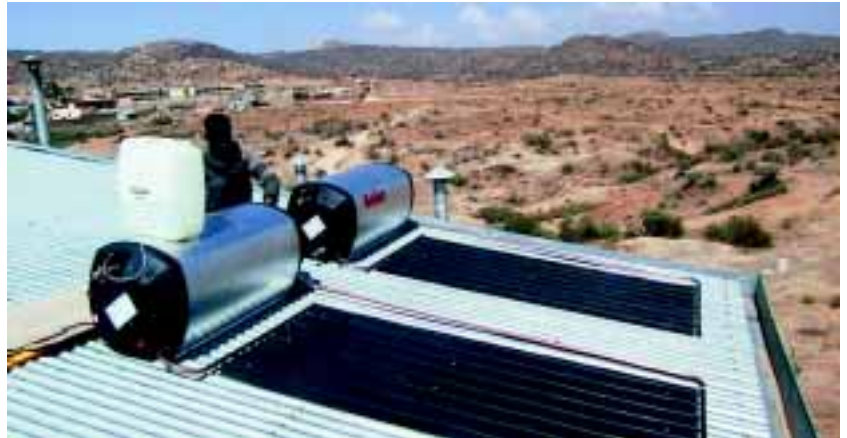
Photos: Hot-water solar installation on the roof of Dekemhare hospital and building of a solar collector.
