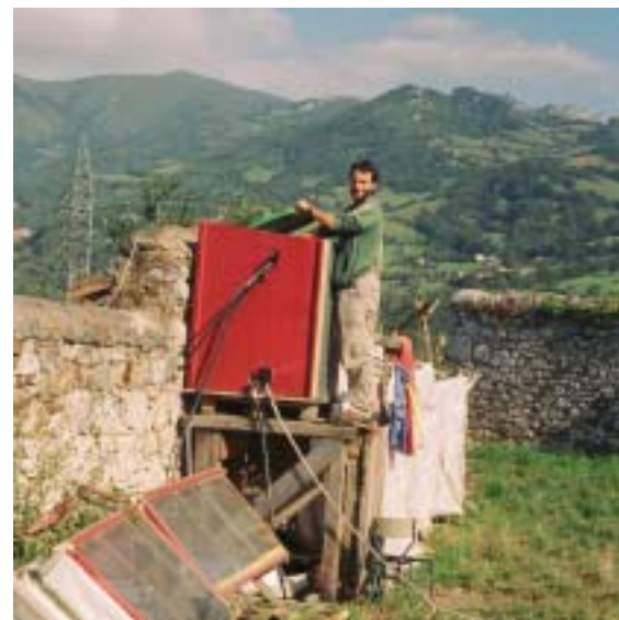
Simple solar heaters provide hot water for showers for the Escanda team
