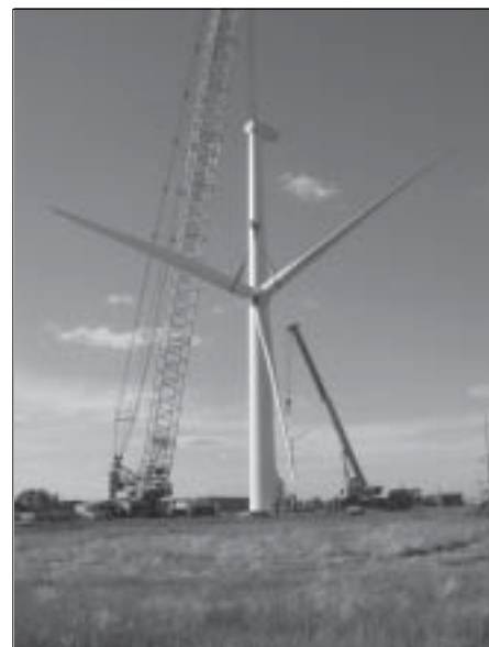
Installation of the wind mills in Ukraine. Photos by Andrej Konechenkov
