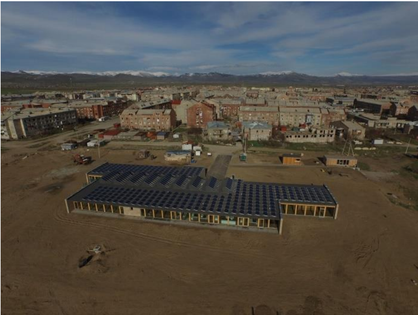
Figure 4. 95kWp PV station in Armenia was installed in Gyumri in 2014 by Caritas Armenia NGO
