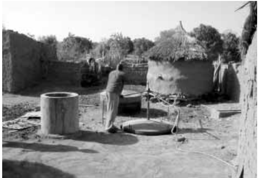
Biogas installation in the village of Konyobla, 30km outside Bamako, Mali's capital
