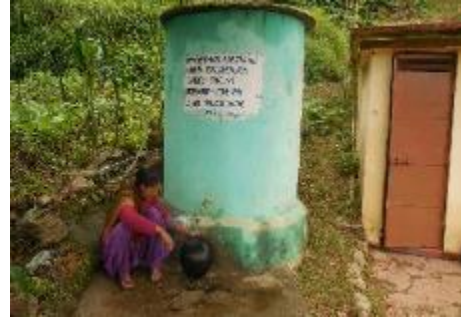
Rooftop Rainwater Harvesting
