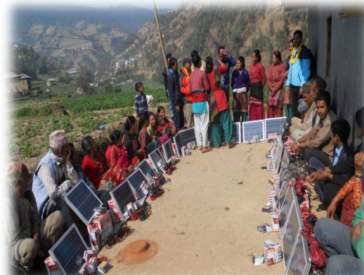
Solar PV Home System
