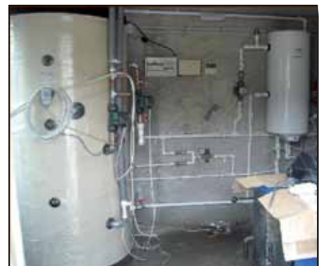
The heating room where you can also follow the heat production of the solar collectors
