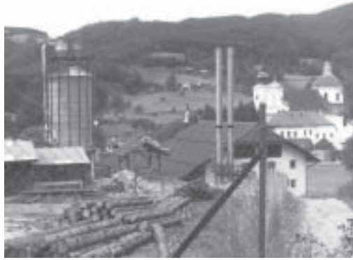
Biomass district heating plant in Slovenia
