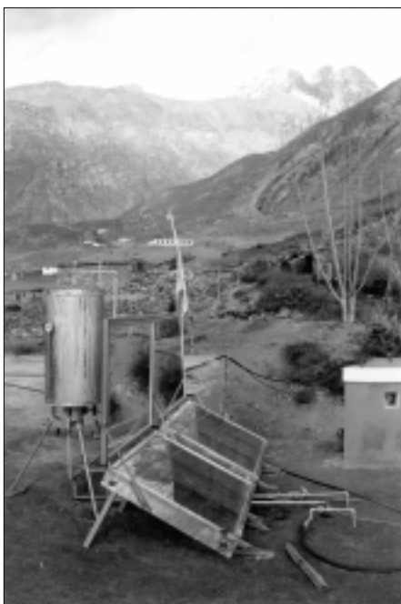
Solar water heater providing a precious service in the harsh climate of this region.
