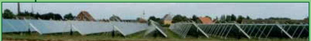
A wind mill park and the world's biggest (8,000 m 2 ) solar district heating plant on the Ærø Island. Photos by Marstal Fjernvarme and Ide Seidelin, Ærø Energy & Environment Office.
