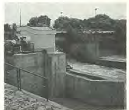
Small-hydro power plant, Slovakia.
