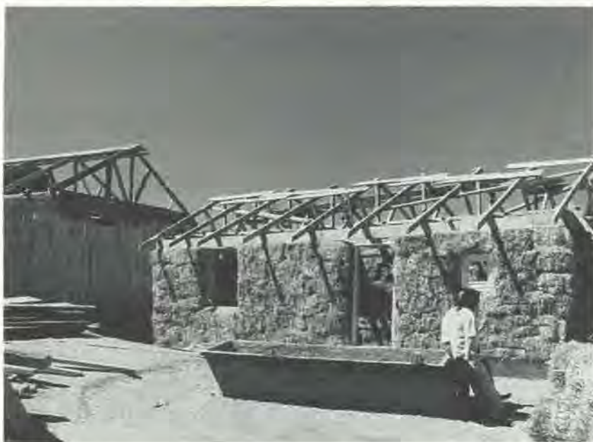
During construction - the super-insulating straw-house in Mongolia.
