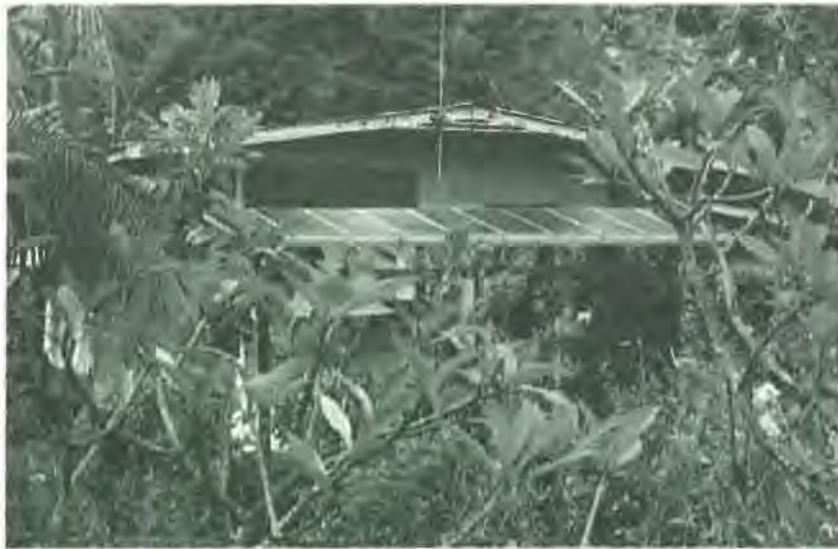
Community solar PV system Polyne- sia, Pacific.
