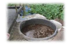
**Bamboo reinforced Slurry Pit**
