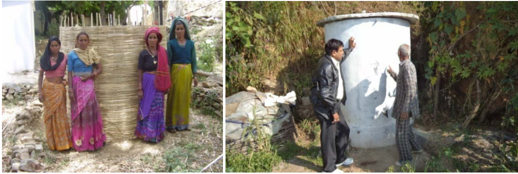
Pictures: Bamboo reinforcement under construction, finished water tank with tap
