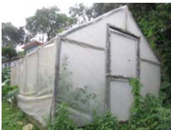
Constructing a bamboo reinforced solar poly greenhouse and growing vegetables in it within the EVD program of INSEDA in India.
