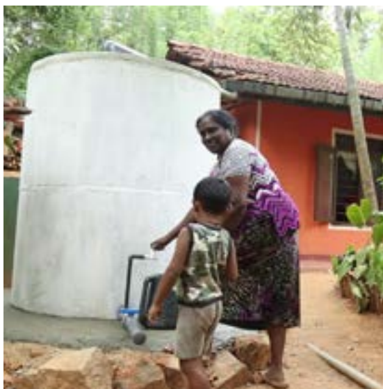
Rooftop rain water tank built from two concrete cylinders in Sri Lanka by IDEA.
