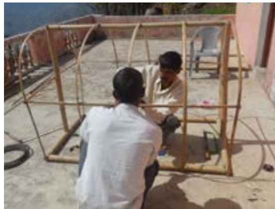
Solar poly tunnel dryer; drying vegetables; and construction of the top part from bamboo.
