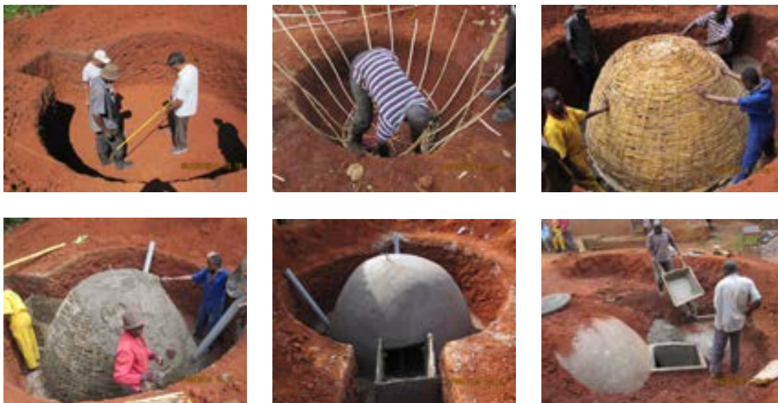
Stages of constructing a household biogas plant.
