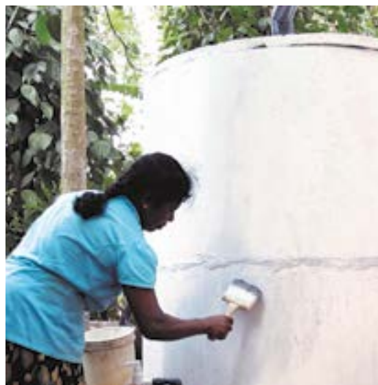
Rooftop rain water tank built from two concrete cylinders in Sri Lanka by IDEA.
