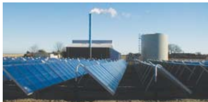
District heating system based on biomass, and solar thermal collectors. Photos by Søren Hermansen, Samsø Energy and Environment Office.
