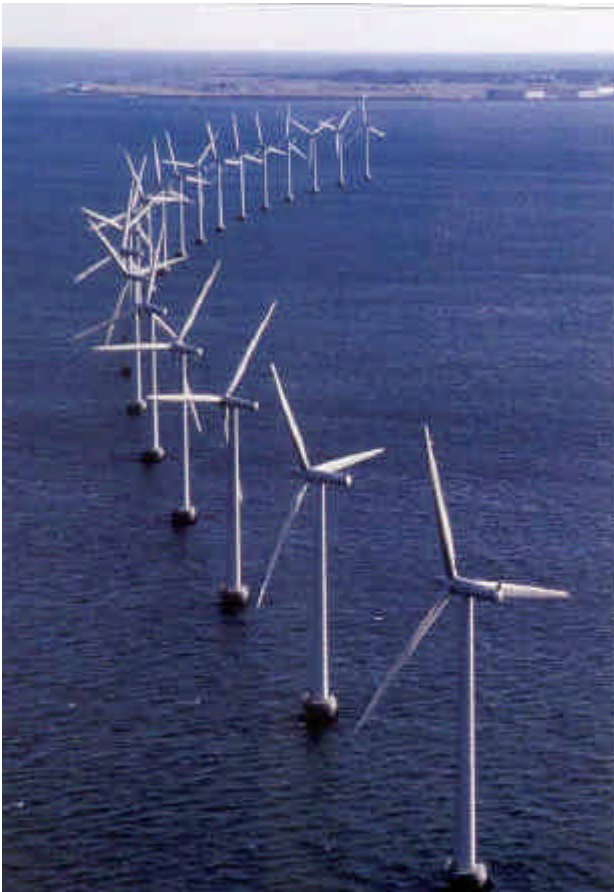
Middelgrunden: The latest and the largest windpower co-operative in Denmark where more than 7000 members own half of this 40 MW off-shore windpark outside the Copenhagen harbour. The other half is owned by the utilities. It was inaugurated in May 2001.
