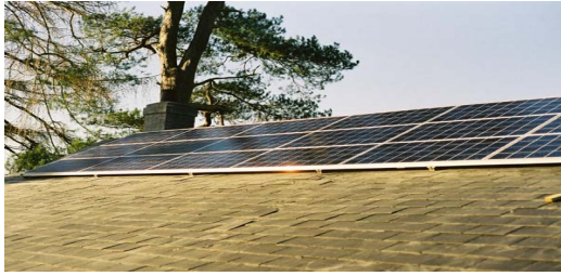
960 Watt photovoltaic array on bungalow at Dolguog, Machynlleth Property also has ground source heat pump
