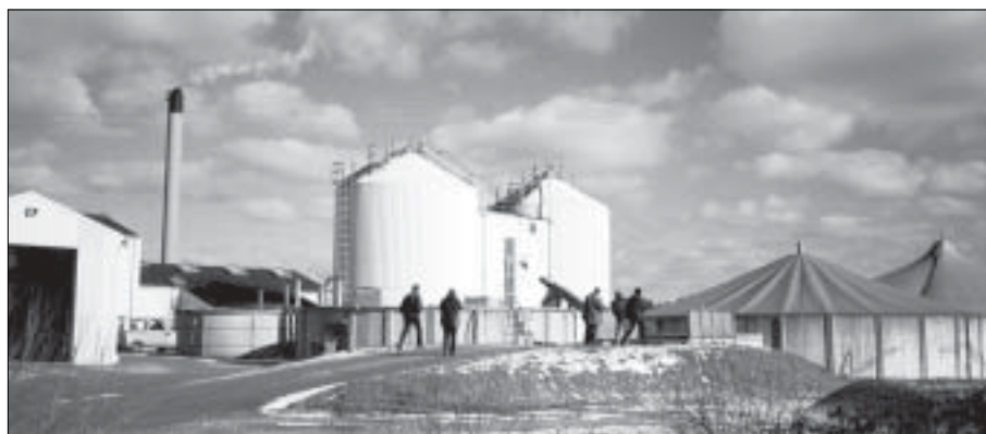
Visiting a biogas plant in Filskov during the study tour in Denmark. The plant receives slurry from 11 livestock farms, and the biogas is powering a 375-kW engine.
