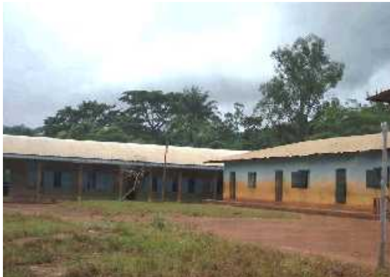
Catholic primary school Bamunkumbit electrified
