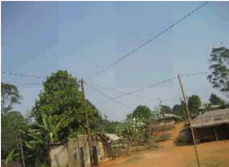
Electrification of Bamunkumbit market
