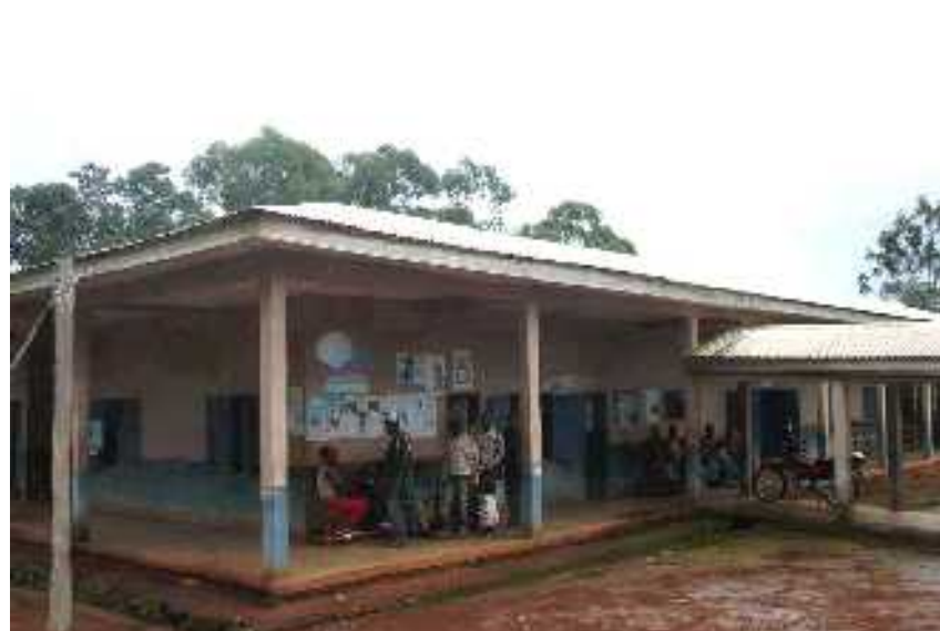
Bamunkumbit's Health centre electrified
