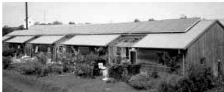
Large, cost-effective solar water heating will be supported by the new directive on energy performance of buildings. Photo by INFORSE-Europe.
