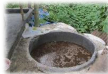
Bamboo reinforced Slurry Pit
