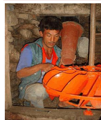
Technician Installing IWM
