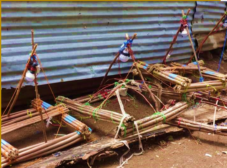
Solar powered lights being used by fishermen in Mfangano Island (Lake Victoria) for the fishing of dagaa (Photo credit: SusWatch Kenya)
