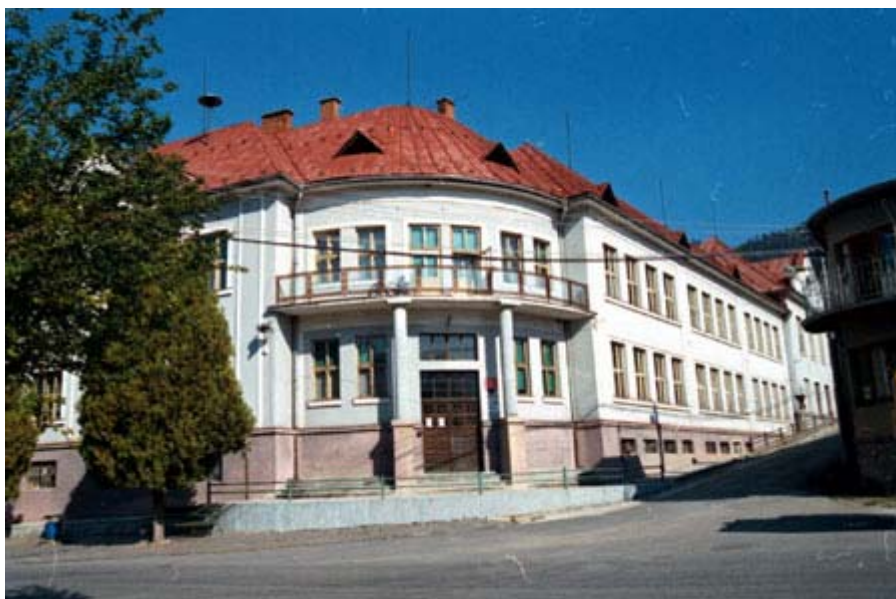
Lubietova: Primary school. Installed output of biomass boiler: 200 kW
