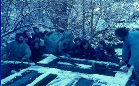
Installation of the CAT hydro turbine
